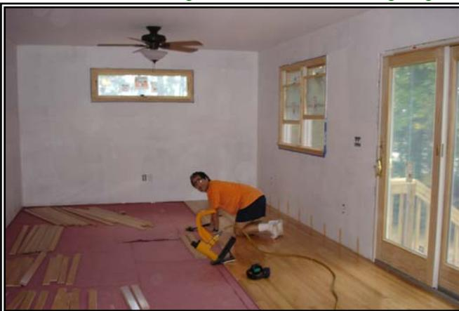
By mid September no more forward progress was being made. I tiled the bathroom. Kim and I installed the hardwood floor. I wired a new circuit for the garage outlets. We painted and I installed baseboard heat and a new zone off of the boiler.
